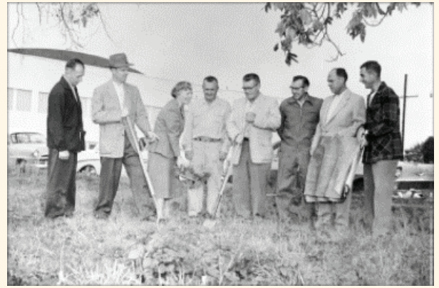
Elsie Stuhr (center) and others breaking ground for THPRD's first building, the Beaverton Swim Center, 1956.
