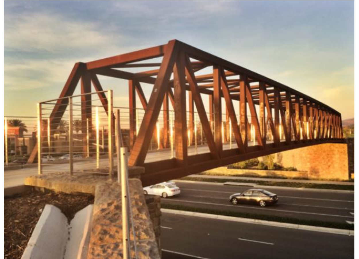
Photo courtesy of Excel Bridge
