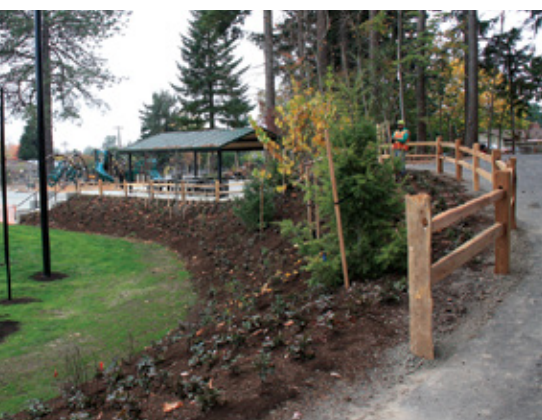
Redeveloped A.M. Kennedy Park features a youth athletic field, ADA-accessible community garden, picnic shelter, play equipment and other new amenities.
