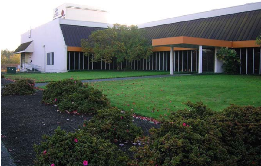
Newly Acquired Maintenance Facility
