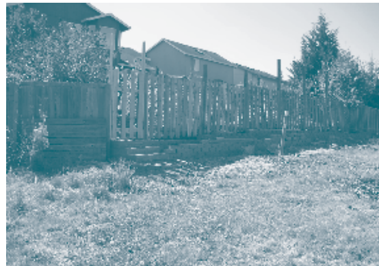
Encroachment into Park District property
