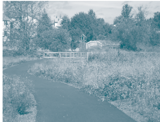
Boardwalk bridge on Rock Creek Trail
