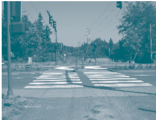
Signalized crossing at 82nd Ave and 122nd Ave includes: 2 marked crosswalks (one for each movement); landscaped median with signal activation; pedestrian push button activation; bicyclist loop detector signal activation; good sight lines; advance warning signs for motorists.
