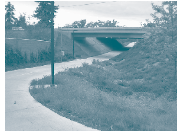
Type 4 grade-separated undercrossing
