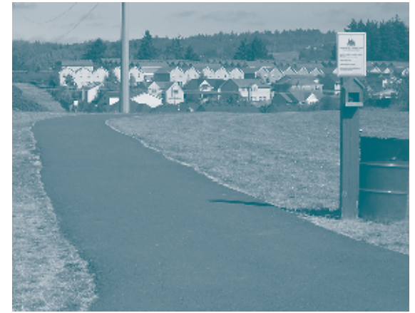
Posting trail operations signs and trash cans improves trail safety
