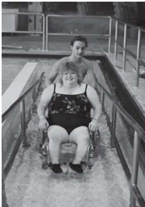
Figure 6-6 A water chair and a ramp or a zero-slope entry can facilitate entering and exiting the pool for a person with impaired mobility.
