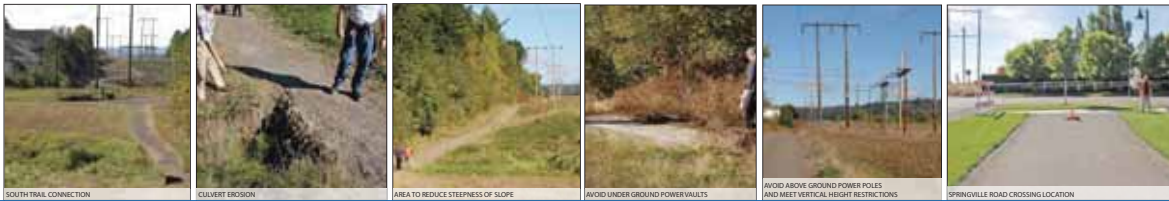
EXISTING CONDITION PHOTOS
