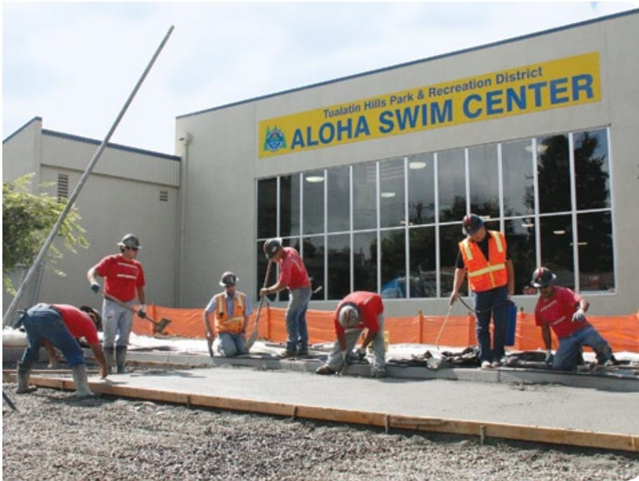
Workers install a new pervious concrete parking lot and sidewalk at the Aloha Swim Center, one of many sustainable approaches to new projects. Permeable surfaces reduce and filter the stormwater runoff entering local streams.
