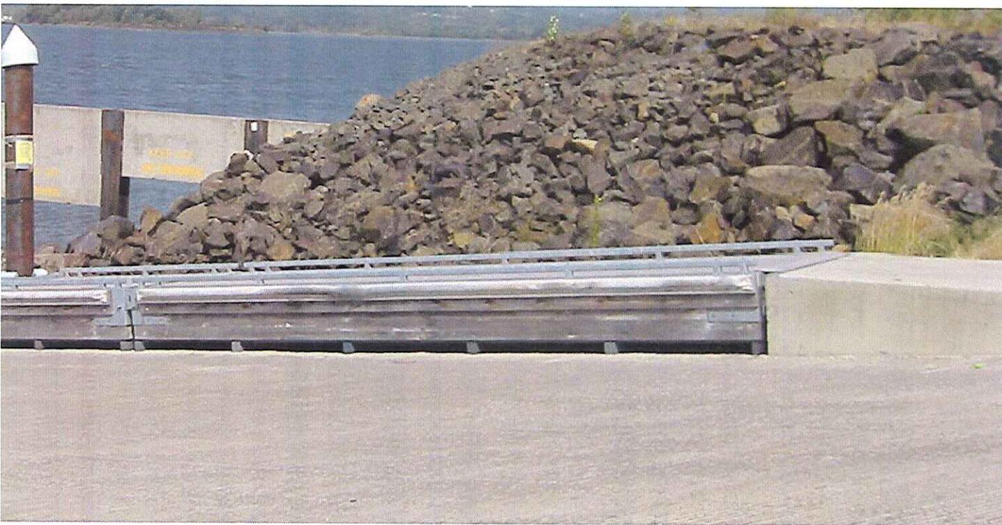
ON GRADE DOCK/CONCRETE ABUTMENT
