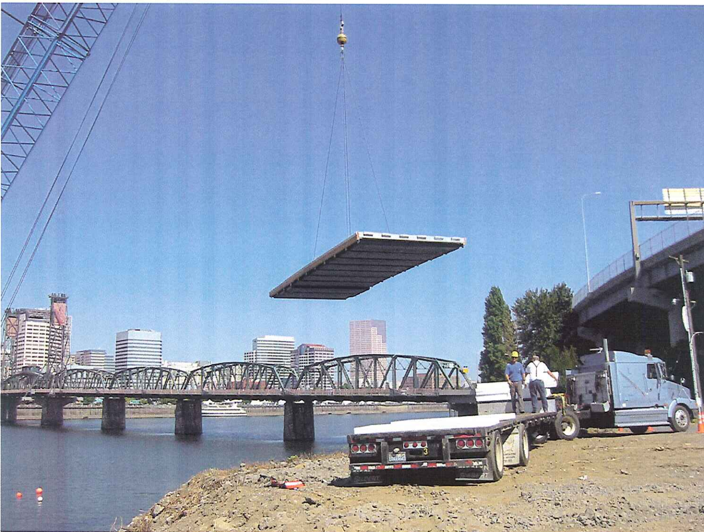
INSTALLATION BY CRANE
