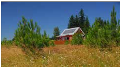
Installed solar panels at Cooper Mountain Nature House
